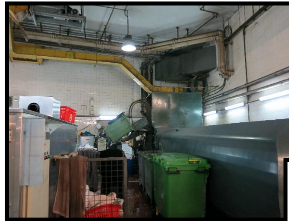
垃圾由翻斗投進固定壓縮機機體 Refuse is transferred into the fixed compaction chamber by the bin lifter or the tipper.
